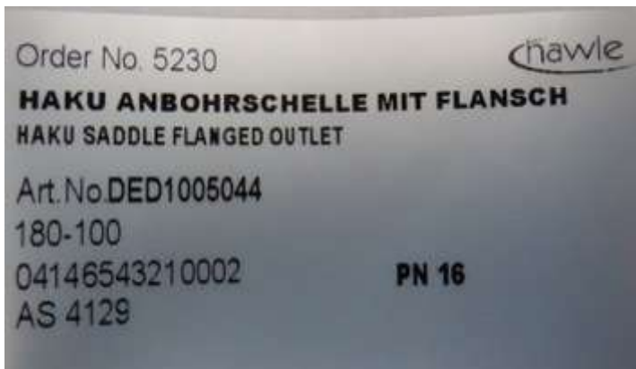
Markings on adhesive label attached to Flanged Off-Take
